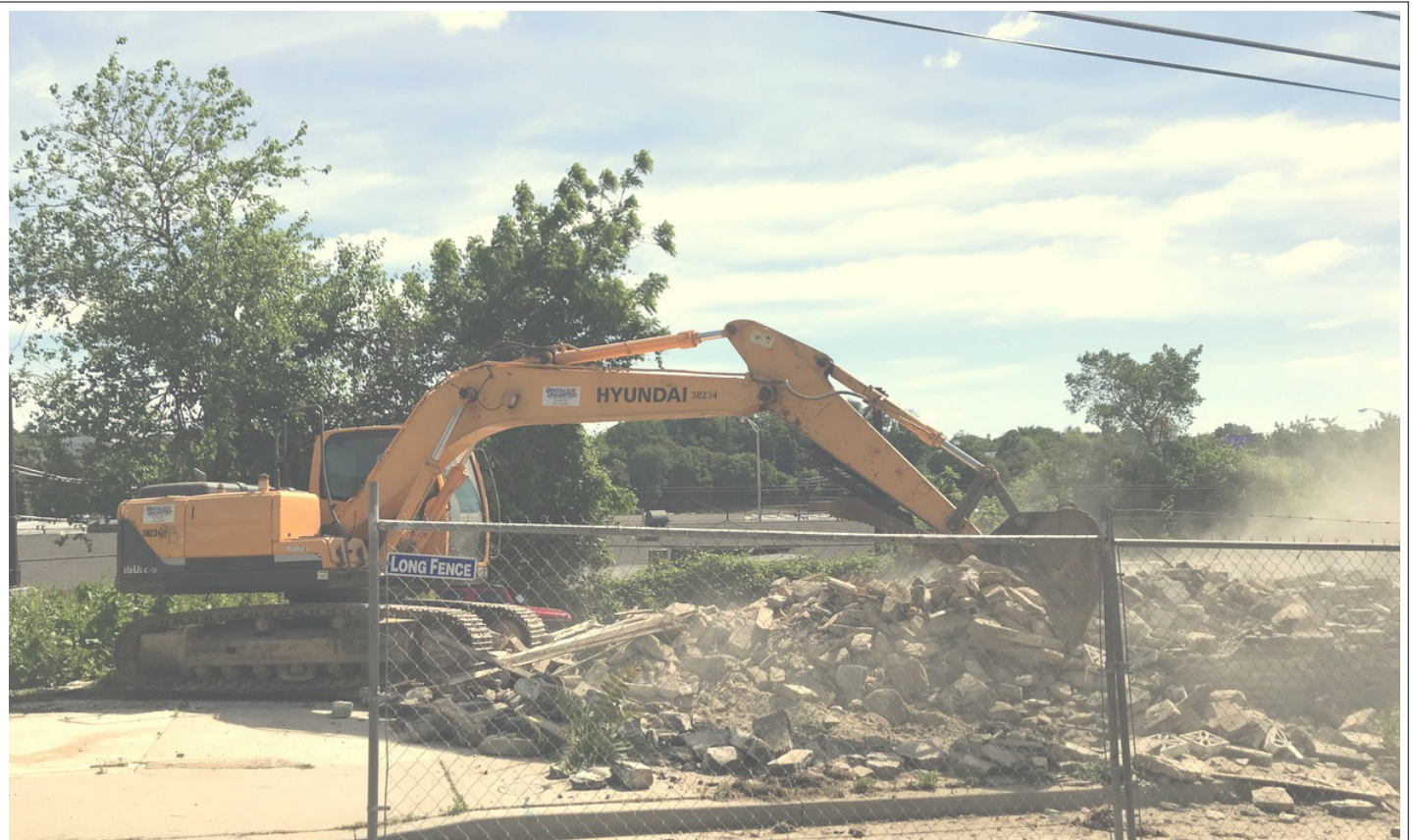
EXCAVATOR TEARING DOWN 35TH CLIPPER ROAD. (MARK REUTTER)
